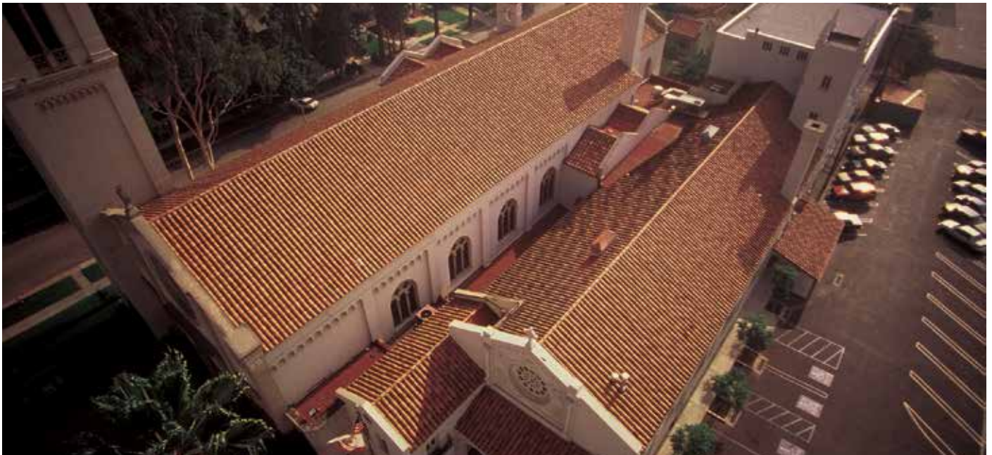
Wilshire United Methodist Church, Los Angeles, CA: Historical Restoration Project: Custom Colors to match original roof tile colors.
