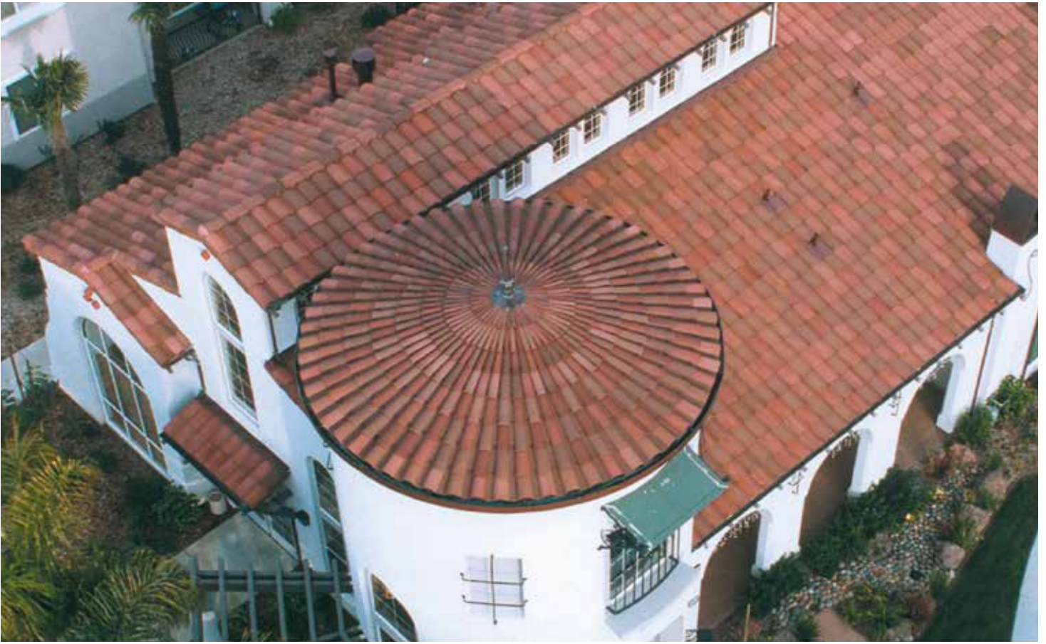
Recreation Center, Turret Tile - F45 Tobacco, F40 Natural Red, 2F43 Brick Red (360° Turret Tile®)
